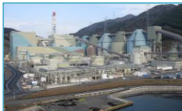
Maizuru Power Station (Coal fired power plant)
